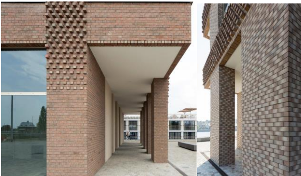
Fig. 7 while in Westkaai towers, the diversity and range of Flemish bricks used in this project allow a subtle color difference between the pair. Tower 5 is yellow and tower 6 red, the classic colors of brickwork, but chosen in tones that make their color highly ambiguous. Using different types of bonds stretcher and English bonds and extruding one of the headers.
