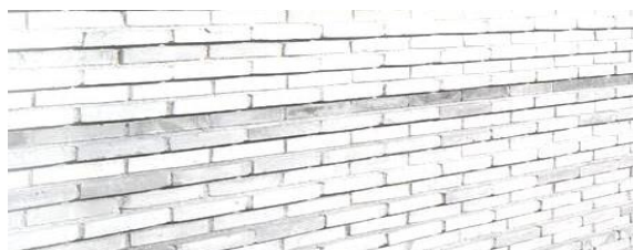
Fig.3 Corbel operation was done by extruding the odd courses. For the whole wall
