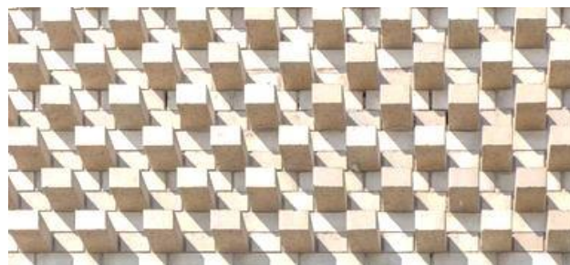
Fig.4 Corbel operation was done by extruding a selective bricks in the wall
