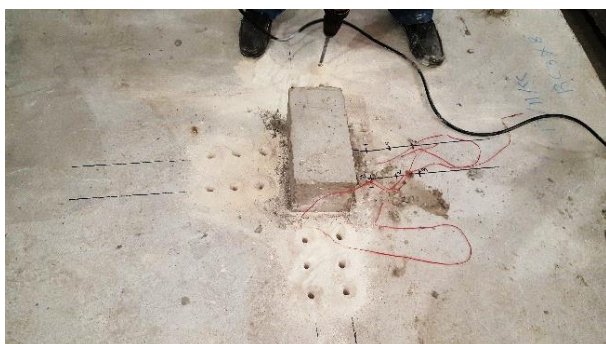
(a) Boring in Slab
