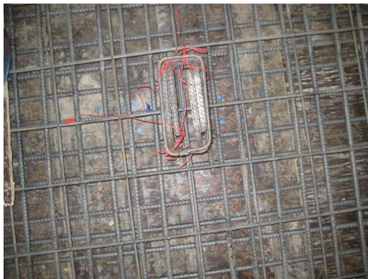
a) Strain Gauges in Bottom Mesh
