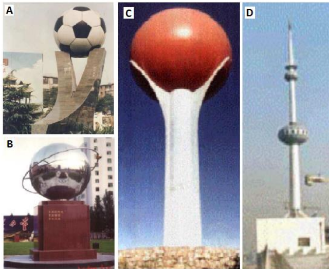
A: a hydrobulged steel football of diameter 4000 mm, B: a spherical vessel of diameter 2.8 m, Landmark of Harbin Institute of Technology, formed by hydrobulging, C: A tower-mounted spherical water tank of 8 m in diameter formed by IHBF, D: Two ellipsoidal communication tower (the bigger one has major axis of 5 m)
