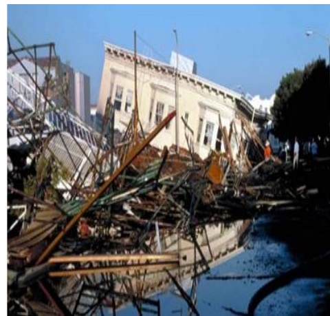
(a) Extensive damage and collapse
