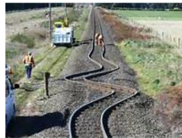
Figure 11 Distortion of railway track
