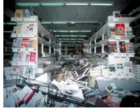
Figure 20 Fallen objects in a book store in Loma Prieta earthquake (Celebi and Brown, 1994)
