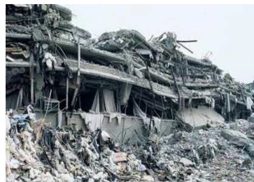
(b) Pancake collapse in of buildings 1985 Mexico City (USGS)
