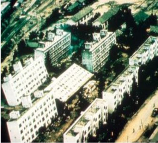
Figure 17 Overturning of building due to soil liquefaction
