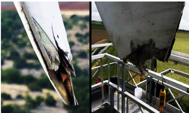
Figure 2: Damaged Turbine Wind Blade due to lightning
