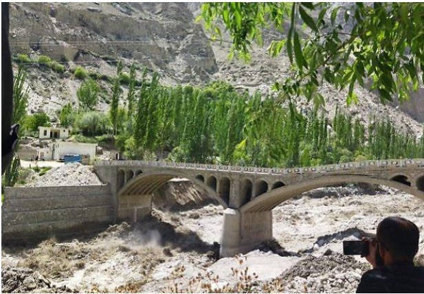
Figure 3 Hassanabad Bridge before Collapse
