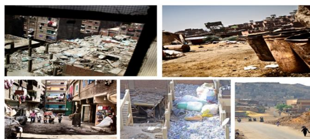
Fig.9 rubbish, Trash on building and streets, un safe entrances, Streets and building
