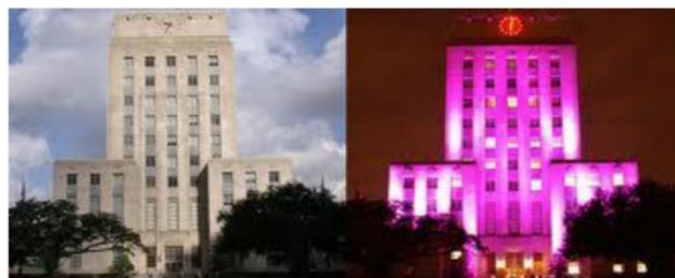
Fig. 5 example for Conventional lighting for historical building
