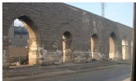
Fig. 4 shows the body of the bridge which consist of about 230 arches
