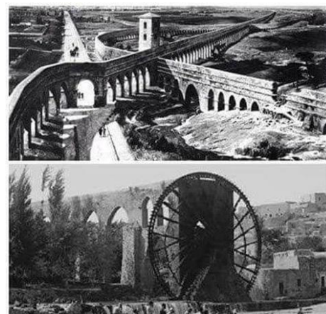
Fig.1 Shows old images for Al O'yoon Aqueduct Bridge
