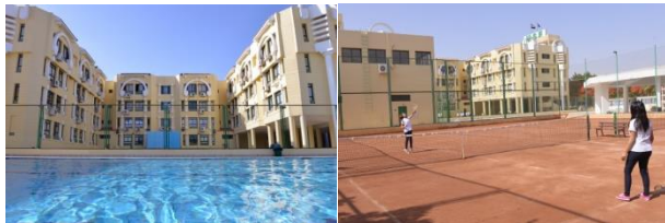
Fig.14. Shows the four floors with a large number of HVACs
