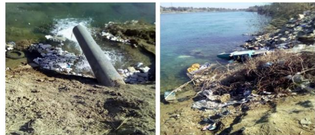
Fig. 3: Drainage and wastes on river.
