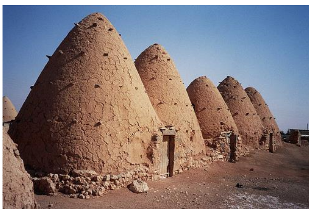
Figure 7: Example for mud buildings where areas have a mud as its raw material
