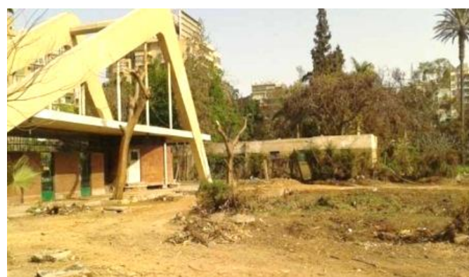
Figure 6: A photo taken at 2017 reviewing the park at time
