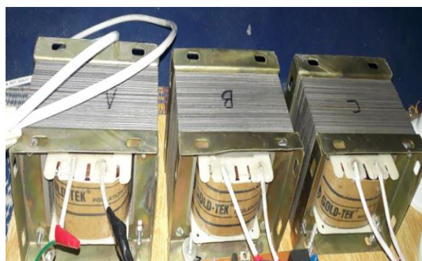
Figure 5 Implementation of Grid Transformer
