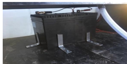
Fig. 3 Battery with mounting brackets used to power the pump
