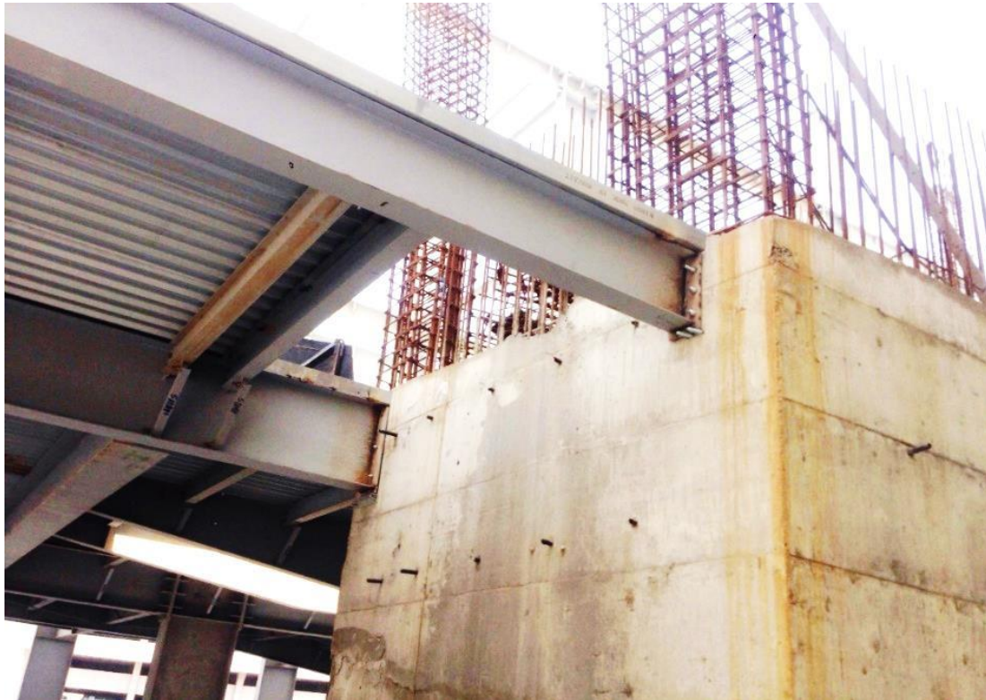
Fig. 1: Examples of Combined Structure in Kuwait
