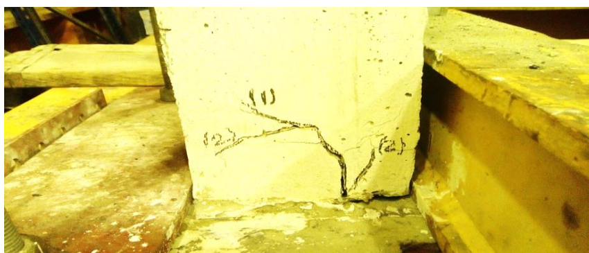
Fig 9: Failure Mode of Frame SC2
