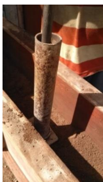
Fig. 10 Manual compaction with steel tamper
