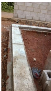
Fig. 7 Construction of kicker for commencement of CSRE walls
