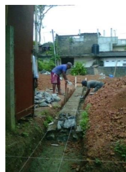
Fig. 5 Construction of foundation
