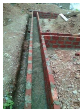
Fig. 6 Arrangement for plinth beam construction
