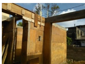
Fig. 14 R.C.C. beam construction with CSRE wall
