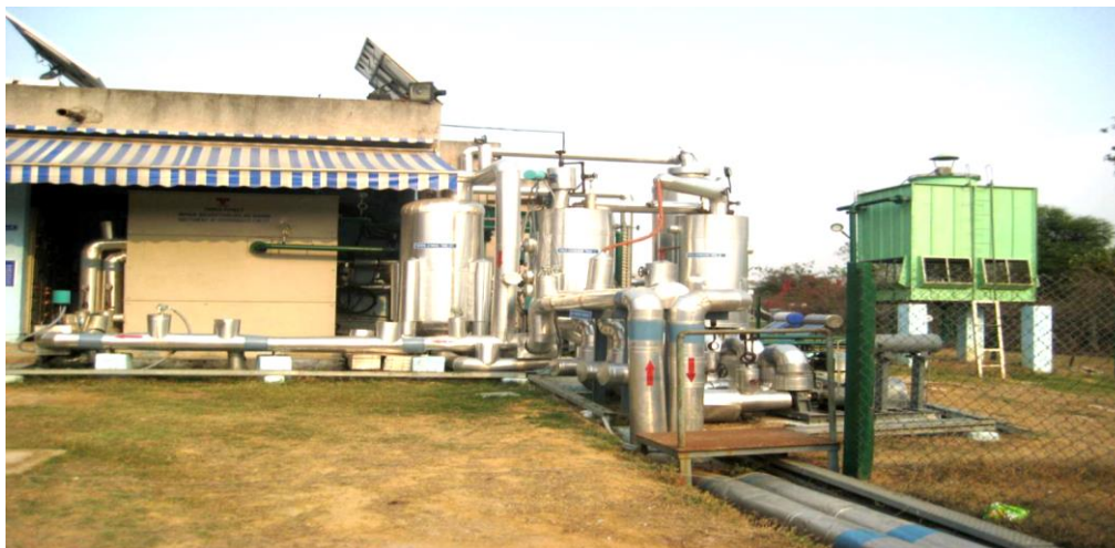
Fig.3 Actual Experimental setup of Triple effect vapour absorption machine at National Institute of Solar Energy
