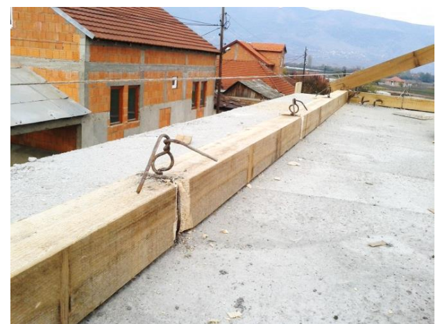
Fig.2 Inadequate anchoring with armature "mustache" and damage to the wedding dress
