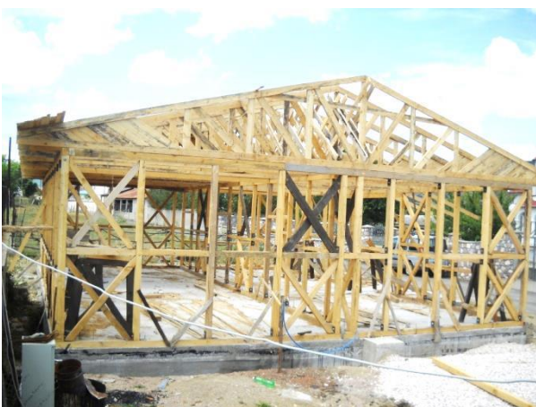
Fig.3 Hinged roofs and skeletal construction in the construction phase before closing
