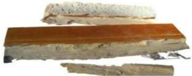
Picture 5: Parquet planks damaged by insects
