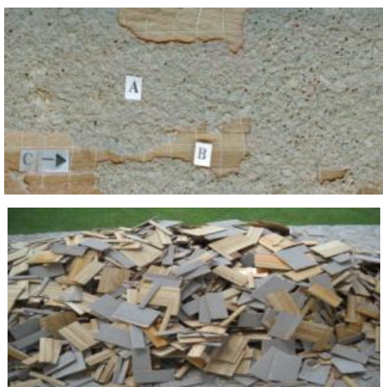
Picture 11: The bottom of the removed part of the parquet (up) and removed lamella parquet attacked by insects (down)
