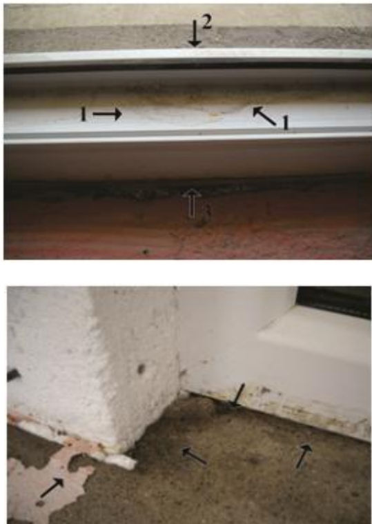
Picture 3: Wetting of the interior spaces through the door (up) and the look of the cement cover under the removed parquet (down)
