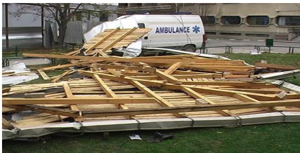
Fig. 2 The roof of the hospital in Tetovo
