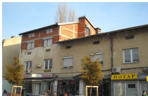
Fig. 1 Changing the height of the existing building by upgrading two new floors
