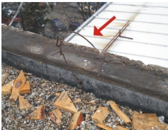
Fig 5. Enforcing the wreath of the roof with armature
