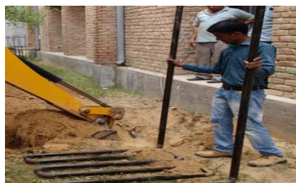
Fig. 4 Installation of Setup Using JCB Machine
