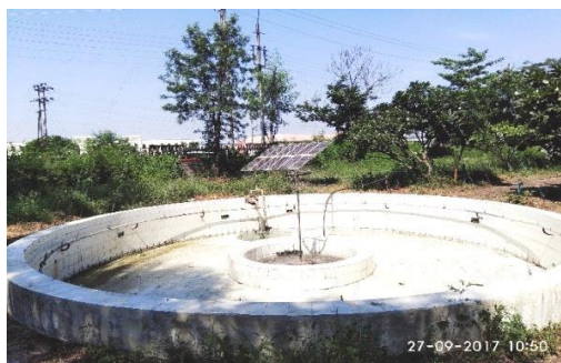
Figure 5 Solar water fountain installed at UTD RGPV
