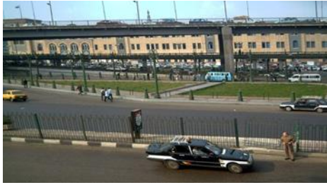
Fig.5 Egypt Railway Station
