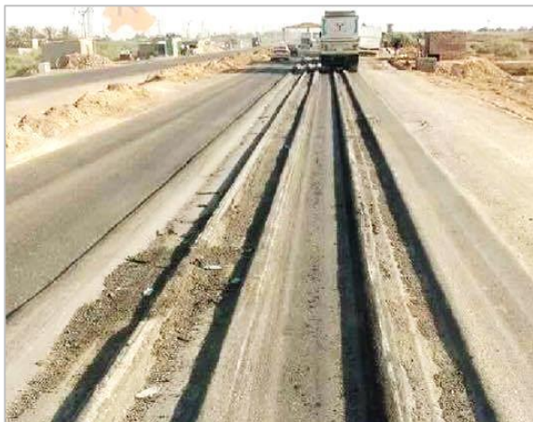
Figure 1: Rutting in Flexible Pavement near the Checkpoint
