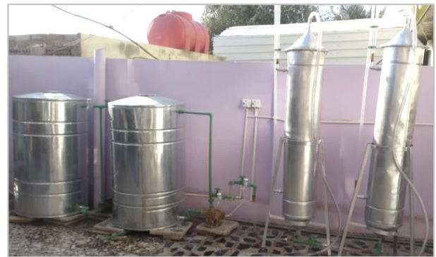
Fig. 6 Photo of the UREL pilot plant
