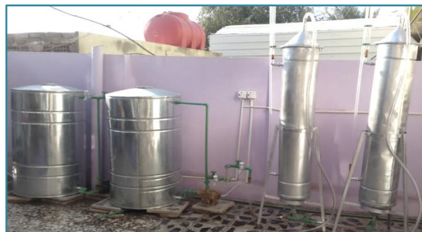
Fig. 3 Photo of the UREL pilot plant
