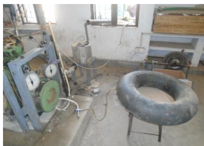
Figure 3.4 Air compressor, Biogas Storage Tube and Its Connection with Engine
