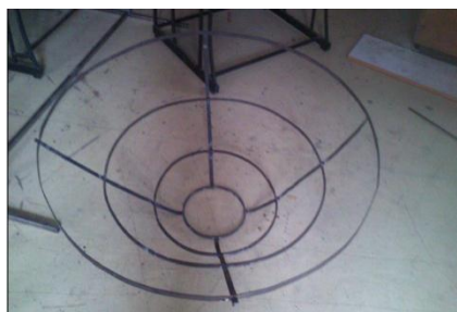
Fig.5 Fabrication of collector frame
