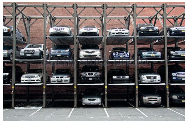
Fig.5 Multi-level car parking (manual)
