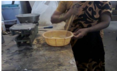
Fig.4 preparation of Epoxy resin
