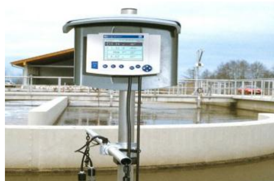
Fig.15 Online Monitoring System
