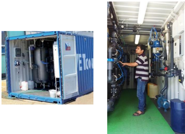
Fig.9 RWT 10 is a Mobile Water Treatment Plant
