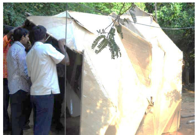
Fig 6.2 Cardborigami structure using card board (Courtesy: Anumapa Kundoo).
