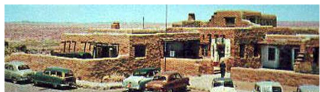
Figure (9) shows the buildings surrounding Petrified Forest reservations in the US.
