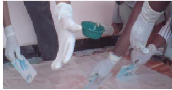
Fig.3 Wetting the cloth with matrix (resin & hardener)
