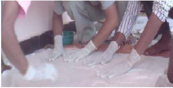
Fig.2 Laying of glass fiber cloth
