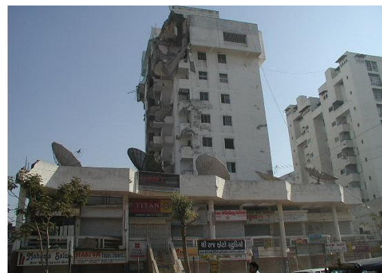
Fig. 1: Failure of R.C. Building with floating columns
