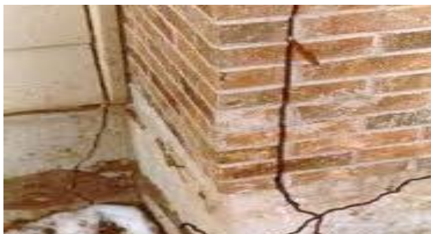
Fig. 3 Vertical cracks on walls due to expansion of soil
