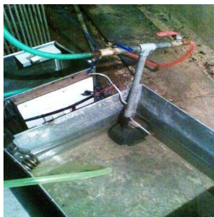
Figure 2.3: Water tank with pump
