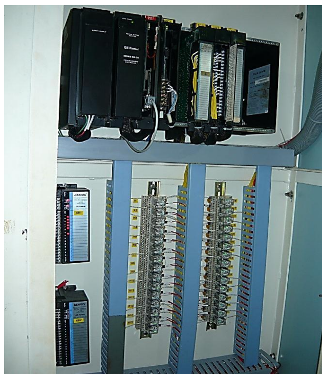
Figure 2 Revamped F&G System
